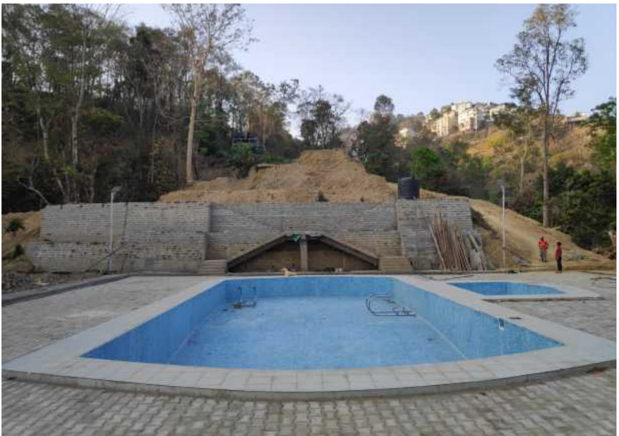
Fig : Development of AMC Eco-Park at Zonaum (Completed) (2016-17)
